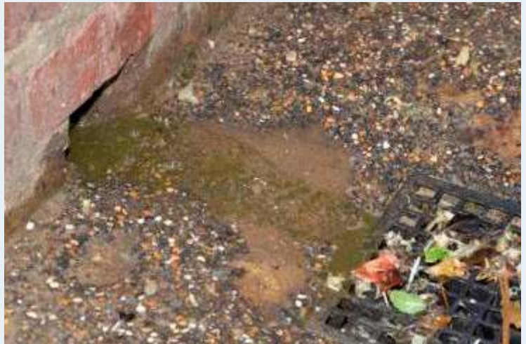
Do not allow run-off to contaminate walkways
